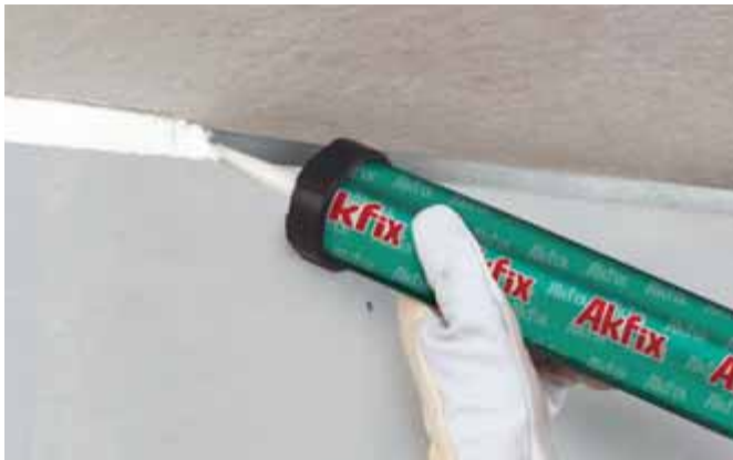
Interior Wall: Fire-Stopping Solution
