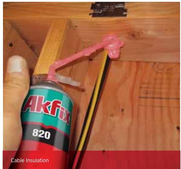
Gap Filling In Duct And Cable Penetration Systems
